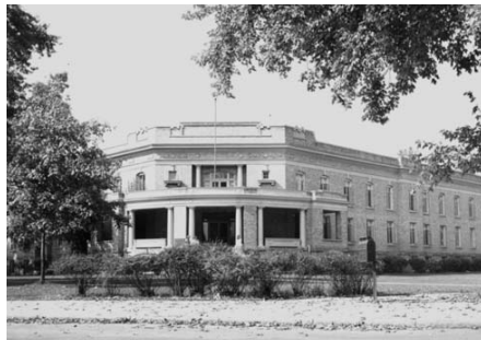
One of the two original buildings on campus, and the first to be completed, Williams Hall has always been at the heart of the academic community at Bowling Green State University.
